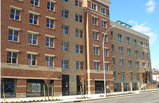
Intervale Green, an environmentally friendly housing development for low income families in the Bronx, New York. Whedco
